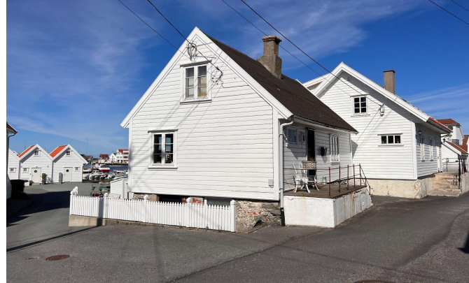
Narrow and disconnected sidewalks
