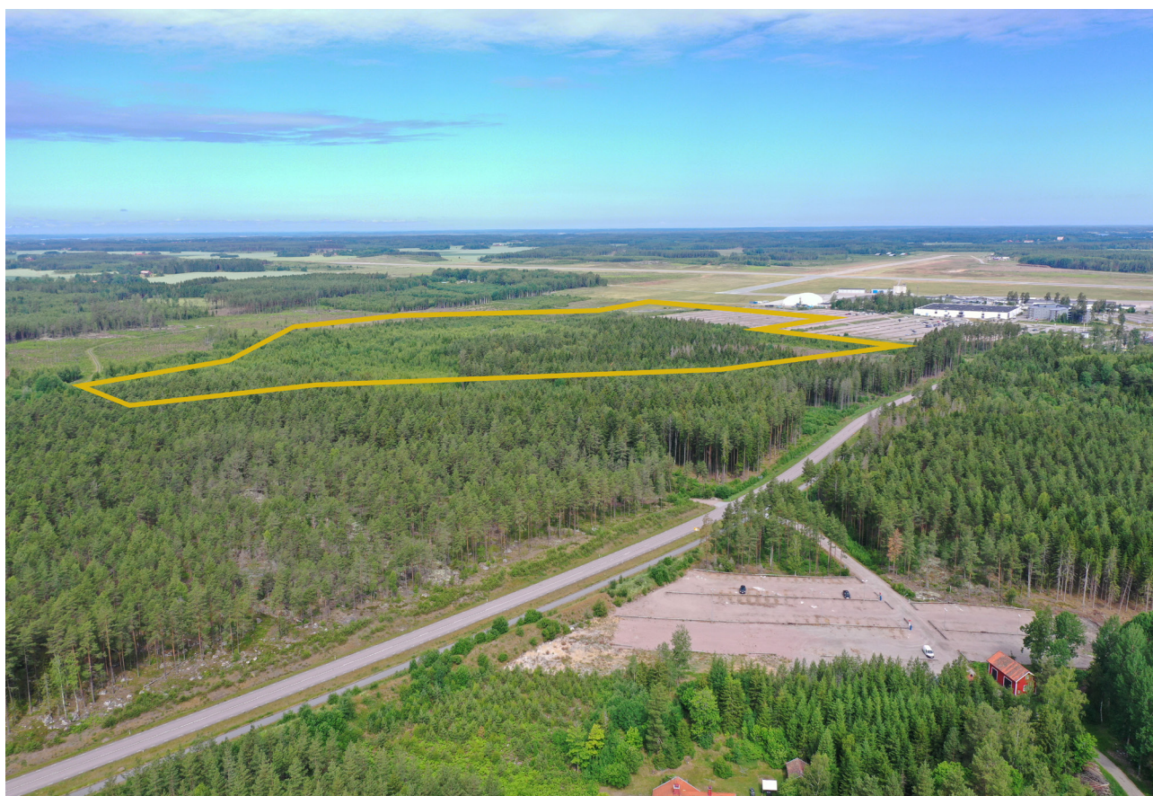
Bird's-eye view over the project site and travel center. Photo by WSP on behalf of Nyköping municipality
