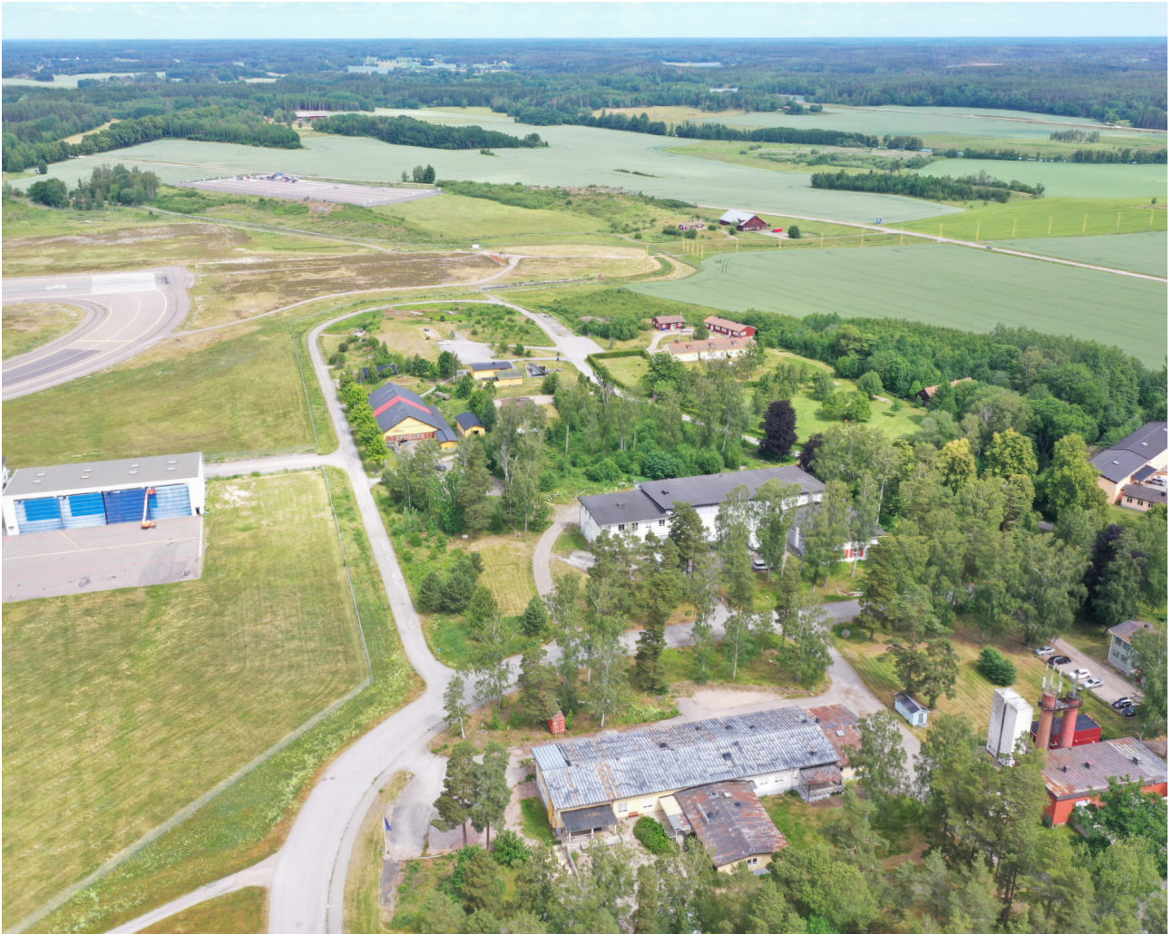
Bird´s-eye view over the F11 area. Photo: WSP on behalf of Nyköping municipality
