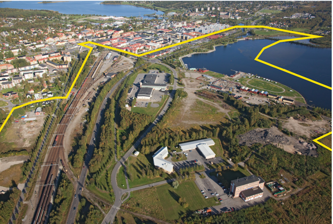
Part of the project site.
