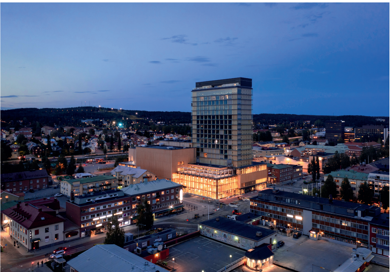
Sara Cultural Centre, built in wood. Photo: Skellefteå Imagevaut.
