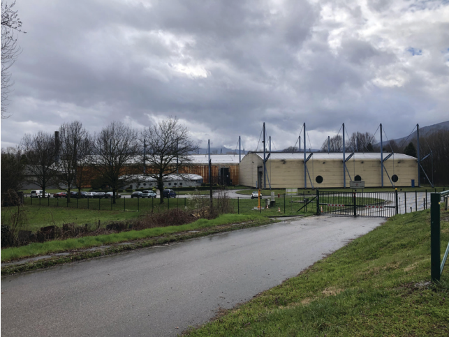
COMPOSTING CENTER OF THE GRENOBLE METROPOLE FR-GAM-C-Po5
