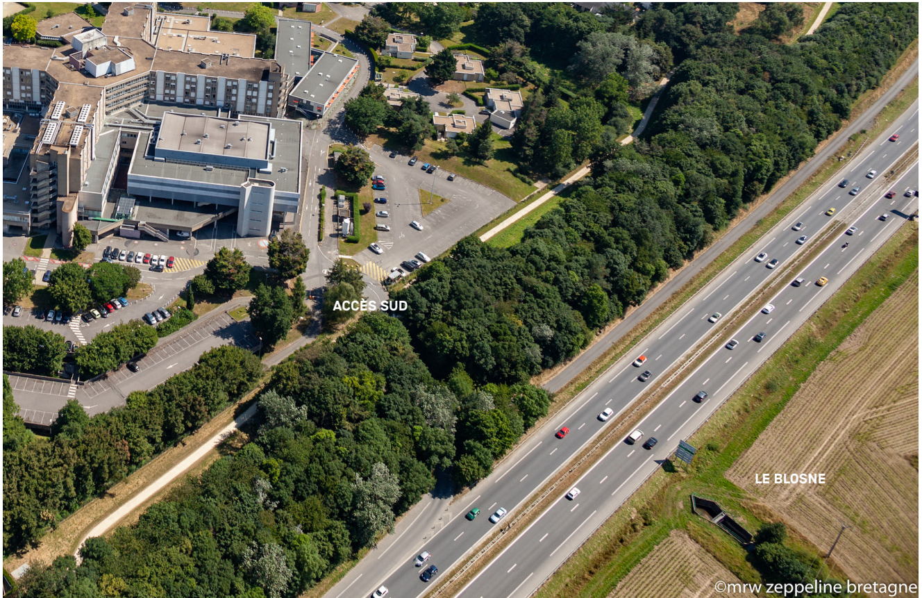
VIEW ON SOUTH RING ROAD AND BLOSNE BURIED PIPELINE FR-RENNES-SS-APo4 © Sabine De Villeroij Juin 2018
