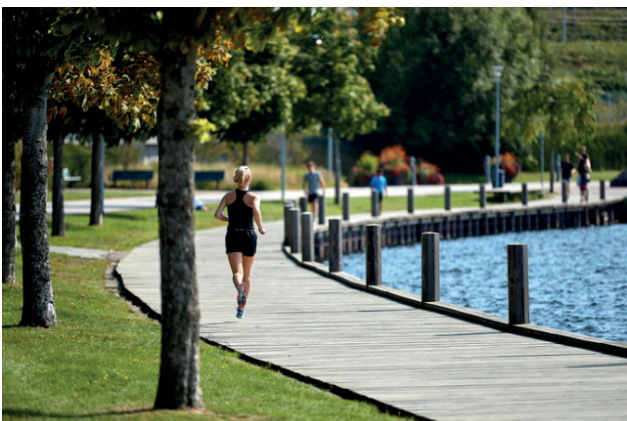
Shoreline boardwalk with stormwater pipes. Photo: Mats Samuelsson
