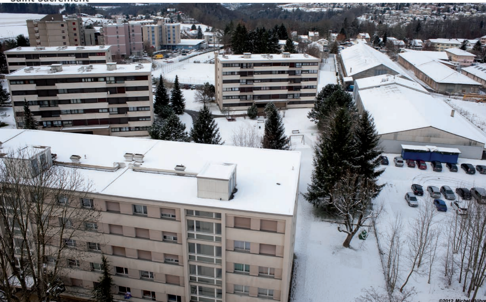
View of the building No. 50, route de Fribourg and of the Saint-Sacrement section from the building at n°33, la route du Centre
