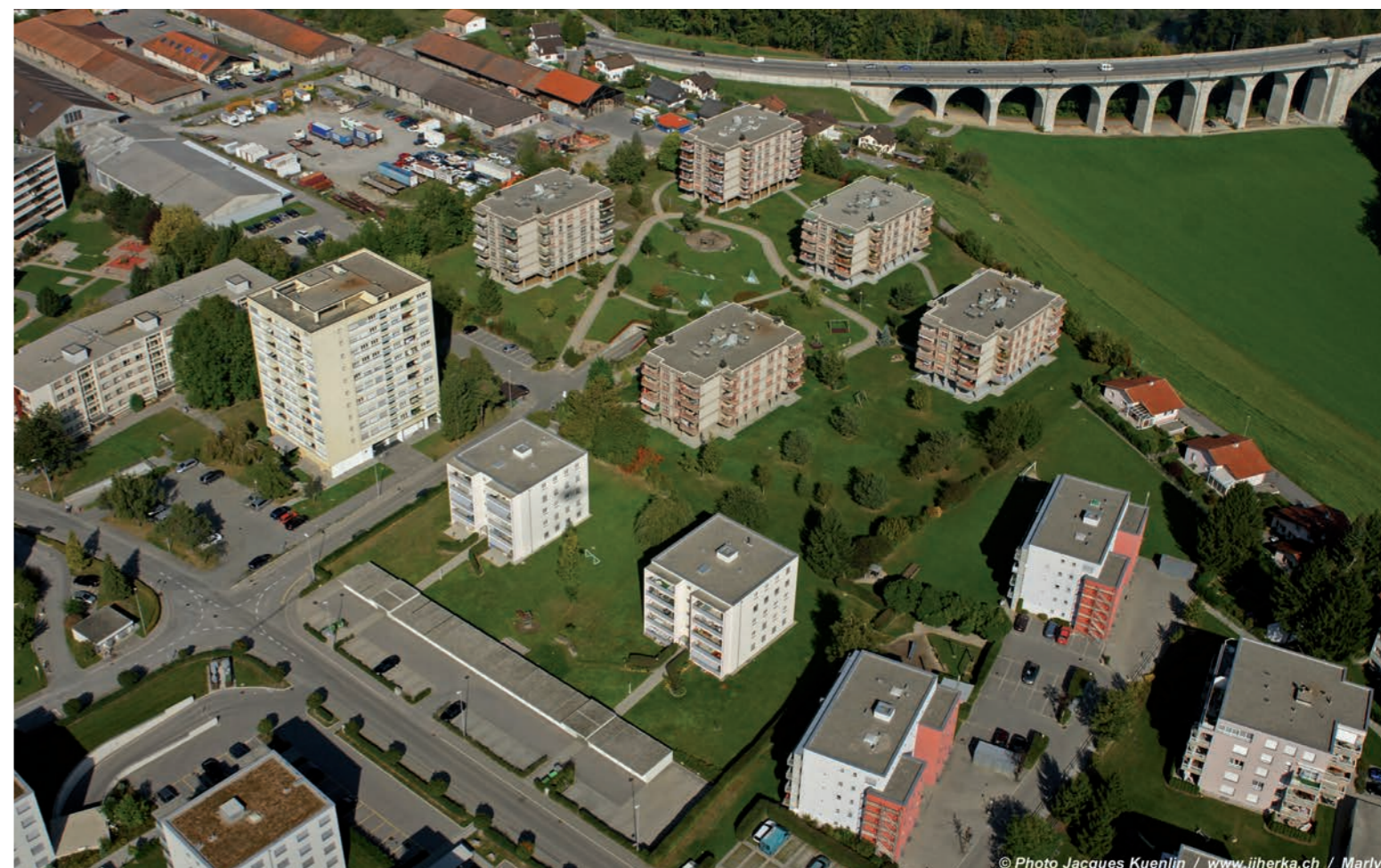
Buildings "route du Centre" in the foreground and in the background the Winckler area
