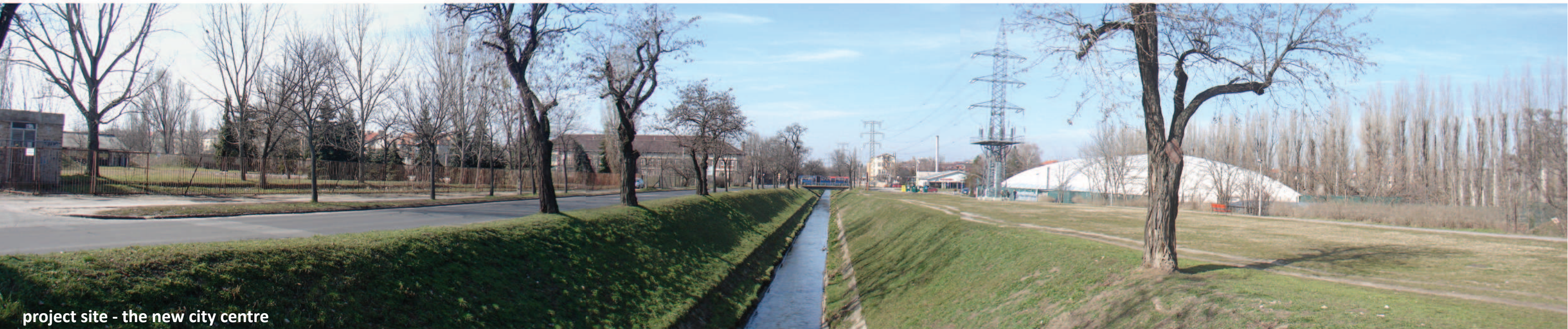
project site - crossing the motorway and the railway yards
