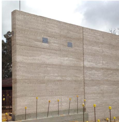
These two elements are mixed with gravel and silt in order to produce prefabricated elements mounted in the concrete structure. The production of the rammed earth walls is forseen to take two months and the curing of each wall, 28 days. A total of two months are forseen for this phase.
