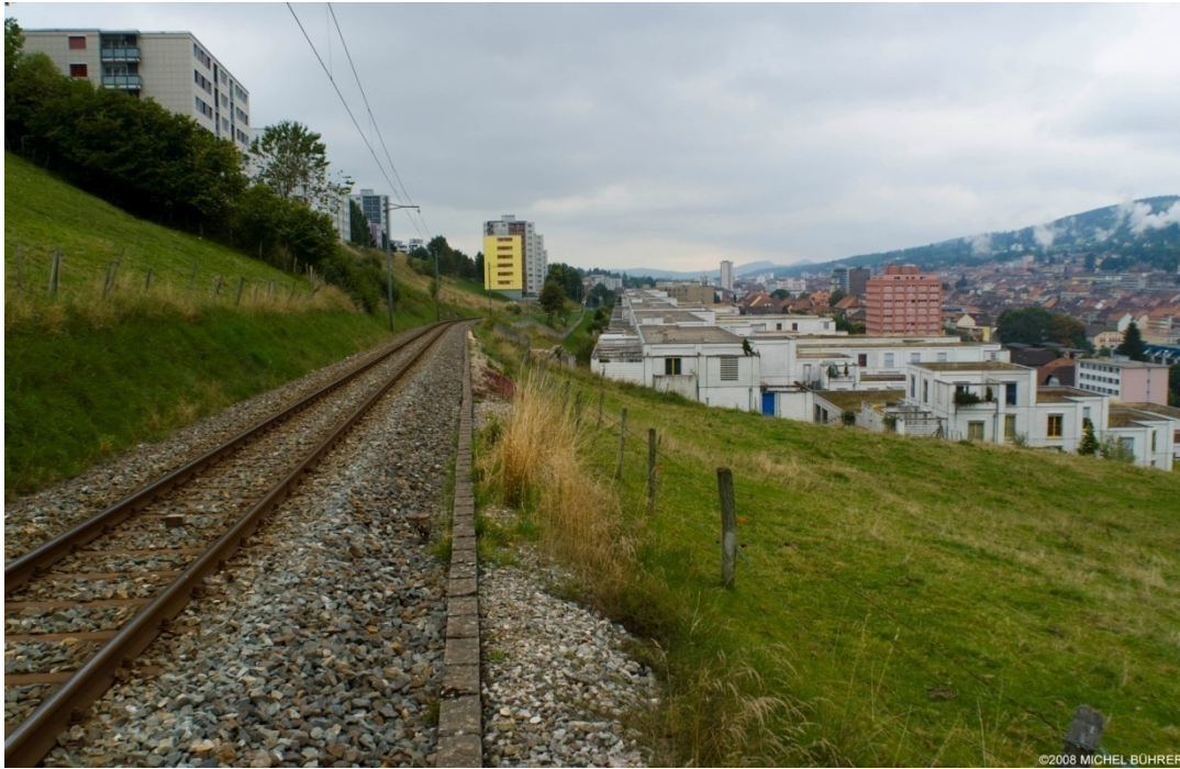
Railway tracks + "Esplanade" district bordering the project site
