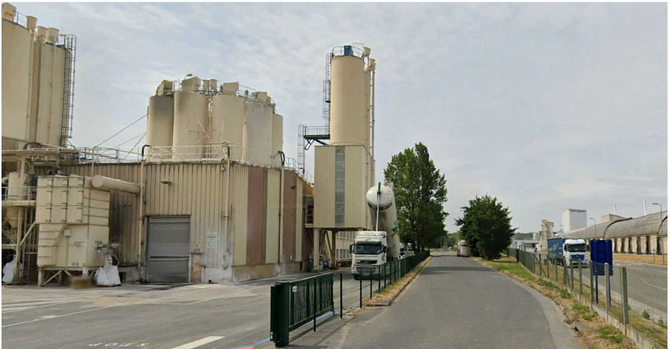
BUSINESS PARK NORTH OF AUNEUIL (RUE IRÈNE CARON) SINIAT (ABOVE) FR-AUNEUIL-SS-P7 SAINT-GOBAIN (BELOW) FR-AUNEUIL-SS-P8
