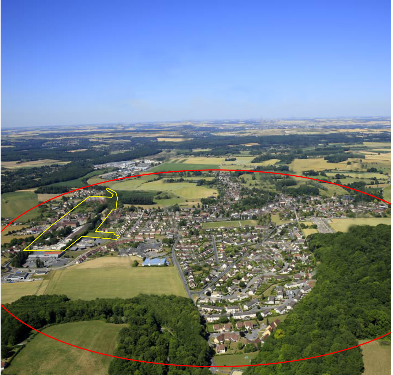
OBLIQUE VIEW WITH THE REFLECTION SITE (IN RED) AND THE STUDY AREA (IN YELLOW) FR-AUNEUIL-SS-AP2
