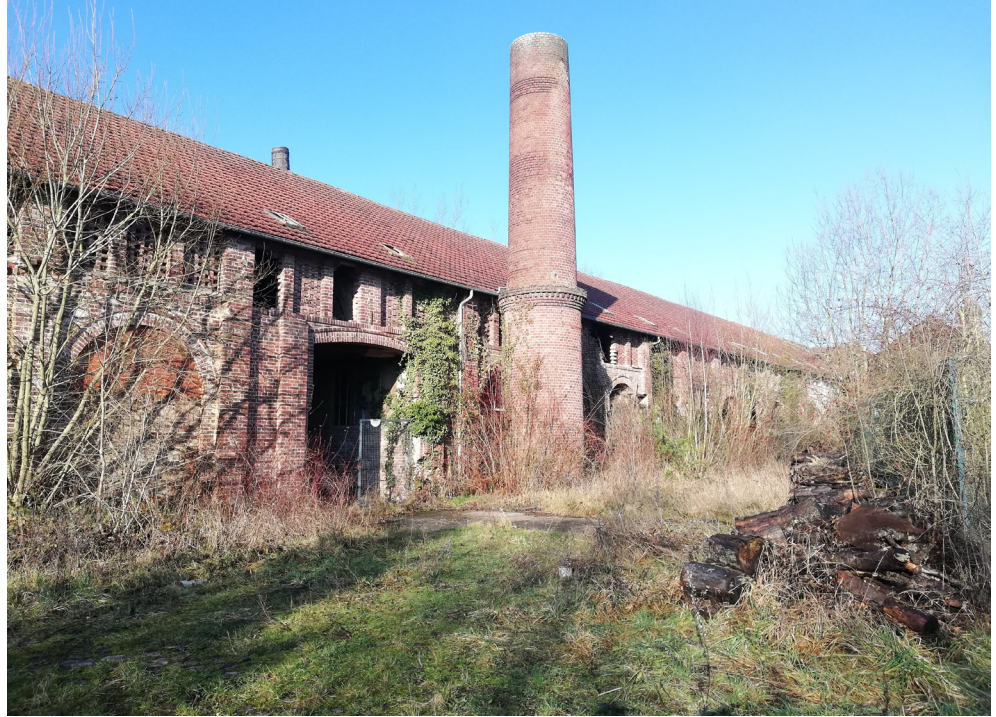
THE OPERATIONS BUILDING OF THE FORMER BOULENGER FACTORY LISTED AS A HISTORICAL MONUMENT FR-AUNEUIL-PS-P3
