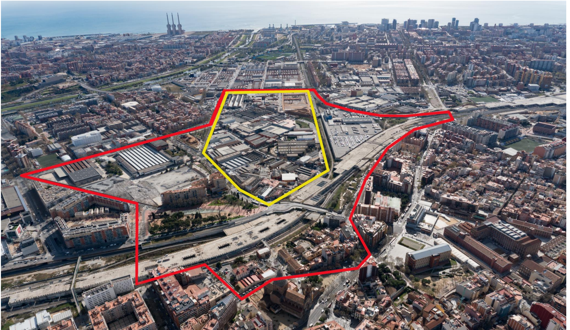
Aerial view of the Torrent de l'Estadella site and its urban surroundings. Reflection Area and Project Area Photography © Barcelona Sagrera Alta Velocidad, S.A.
