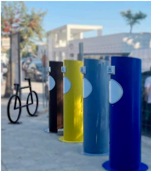
New pneumatic waste collection system - under testing
