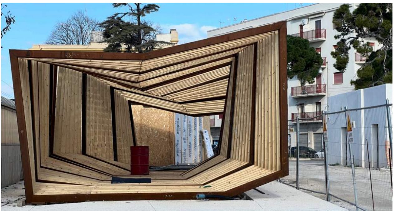
Velostation project nearing completion
