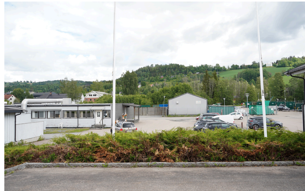
Recycling station at the Lupro site.
