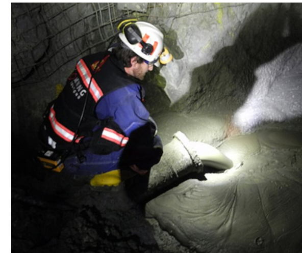
Underground Backfill. Photo: Sika Canada
