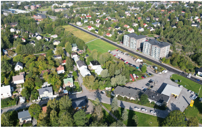
Aerial photo of the middle part of the project site. © Sami Järvelä
