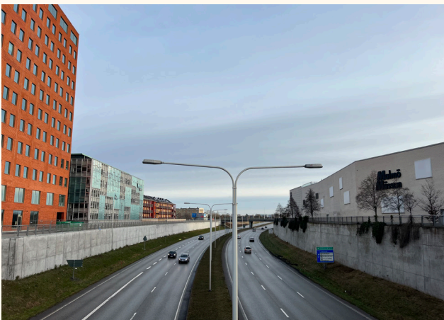
Annetorpsvägen is part of Inre ringvägen, Annetorpsvägen. The section within the project site is prepared for decking. Photo: Emily Evernäs
