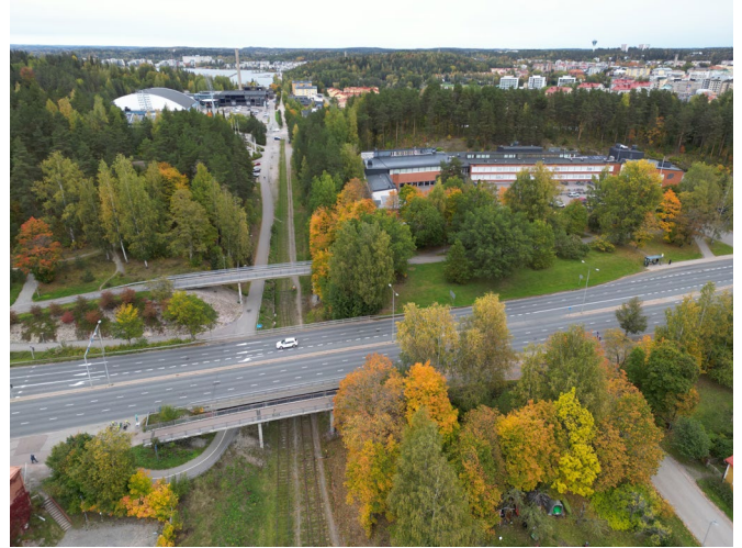
Entrance to the project site and to the lake from the southwest. Salpausselkä comprehensive school on the right. © City of Lahti
