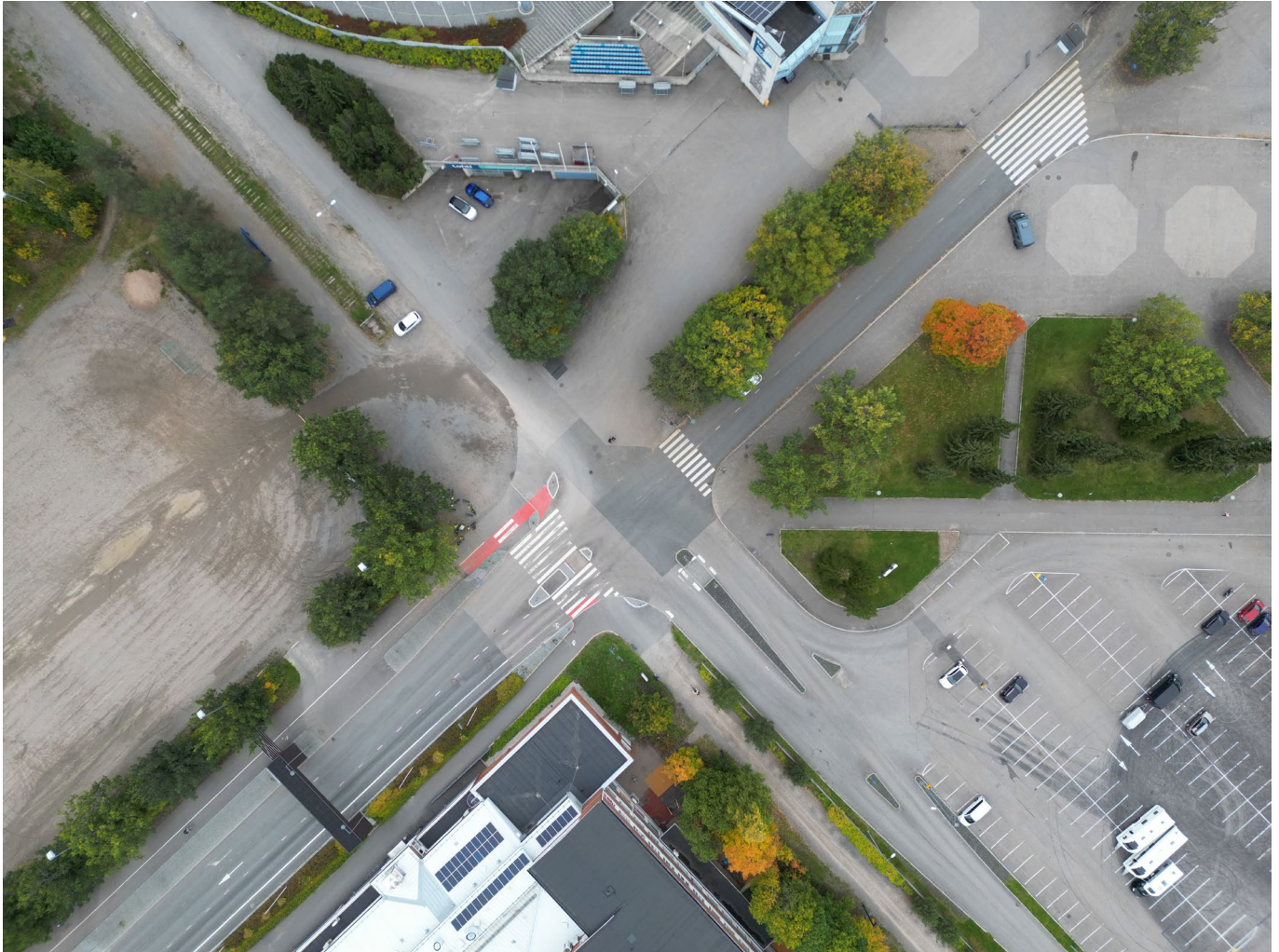
Aerial view of the entrance area © City of Lahti
