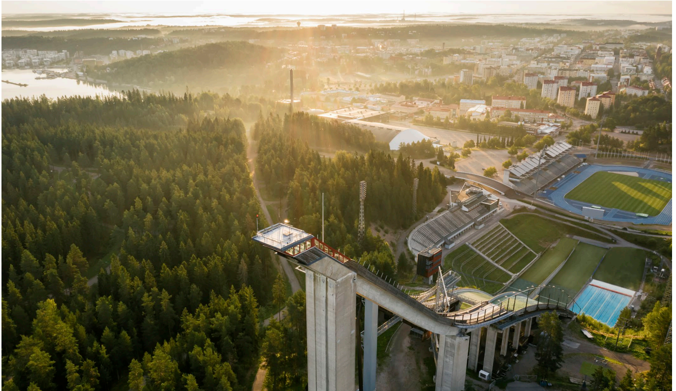
Project site and reflection site from the west © City of Lahti
