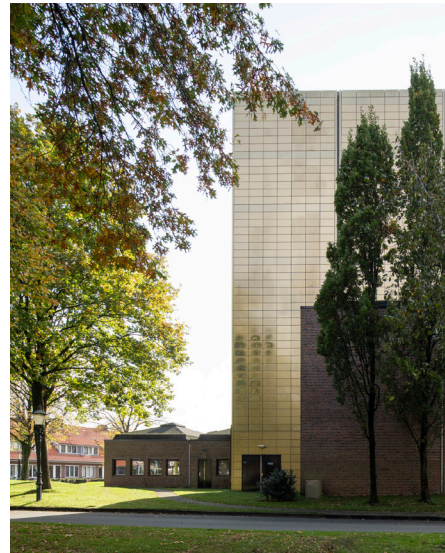
Rear side of the Flint along Plantsoen
