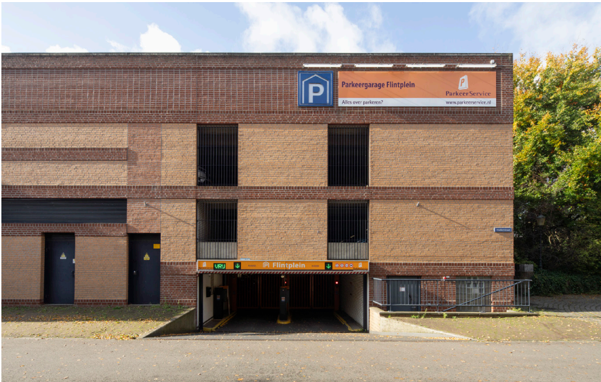
Parking building view from Walikerstraat
