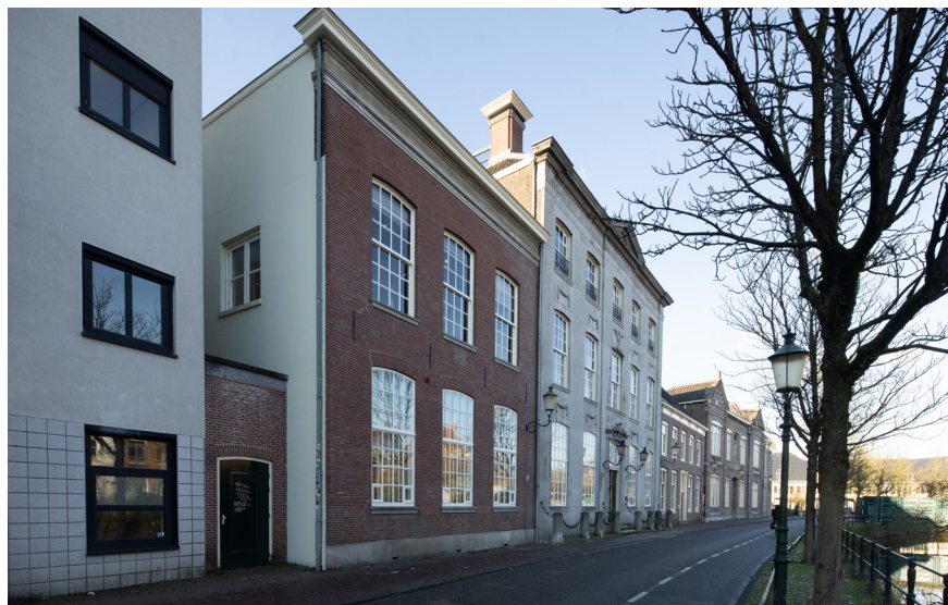
View of the Westsingel street
