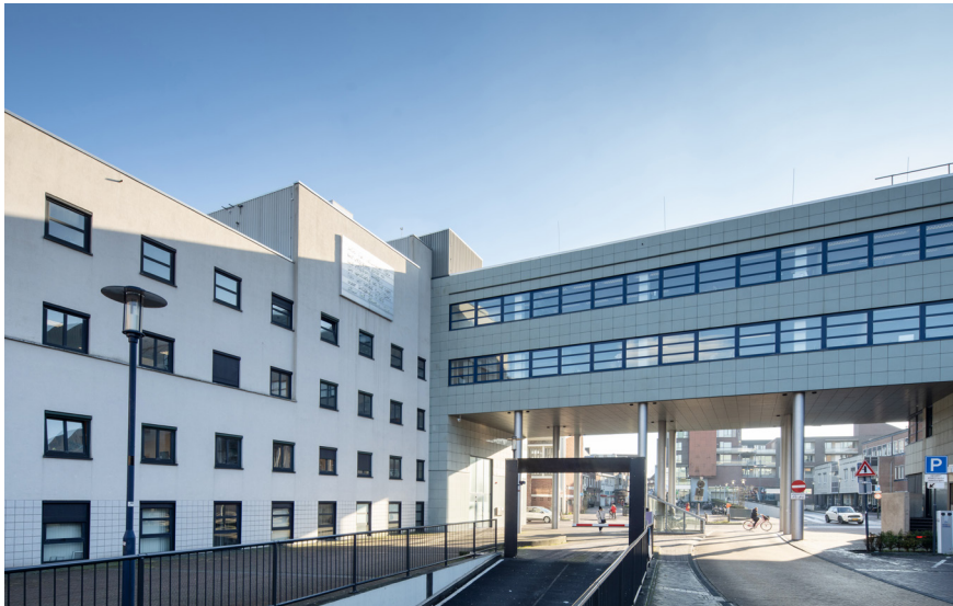
View from Stadshuisplein parking area
