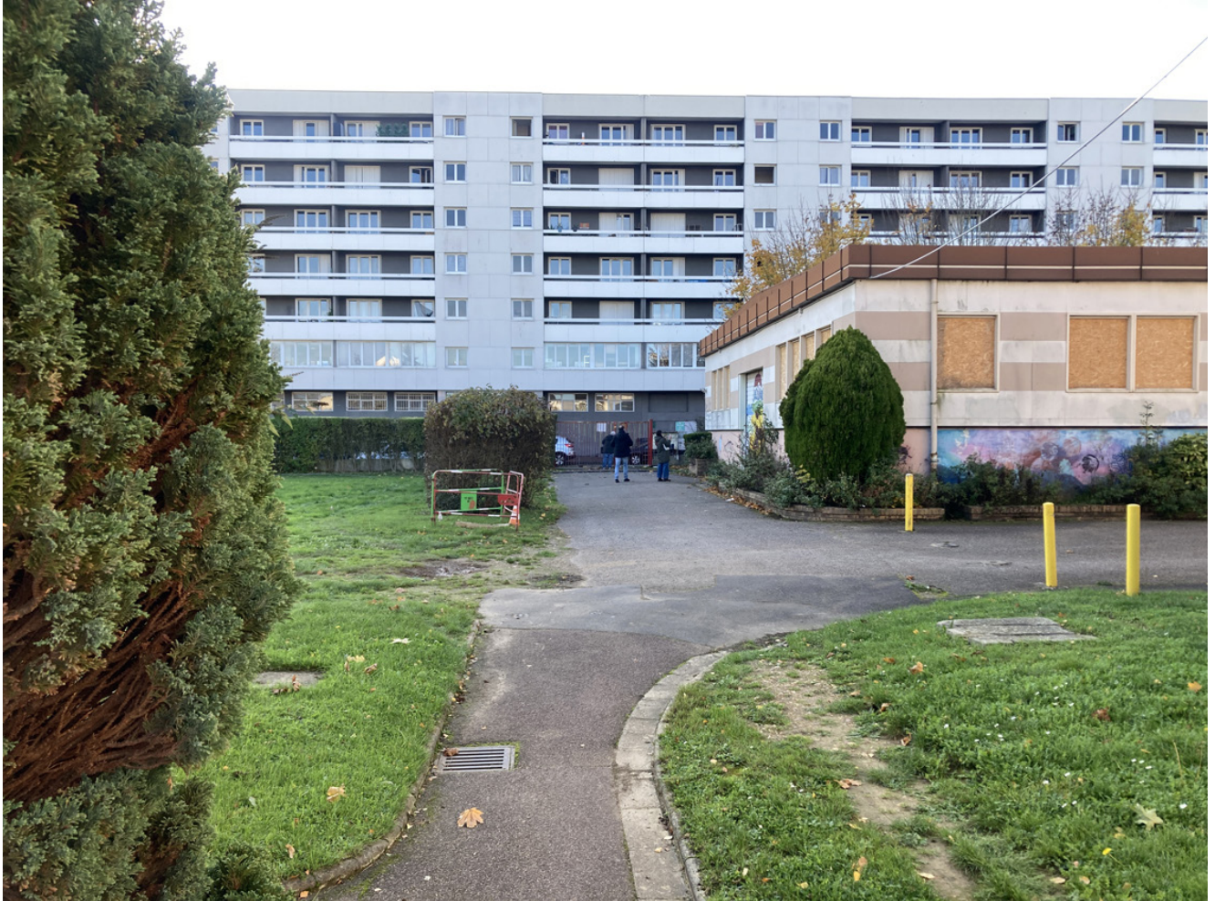
BACK SIDE OF THE MOLIERE'S HOUSING SLAB
