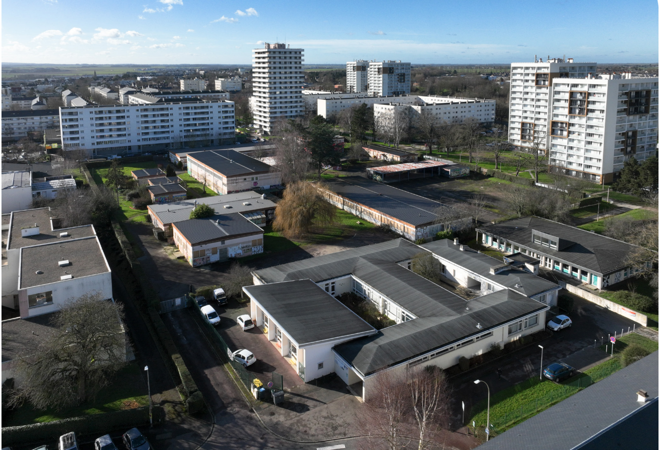
VIEW OF THE ANCIENT COLLEGE'S SITE, TOWER AND SLAB MOLIÈRE
