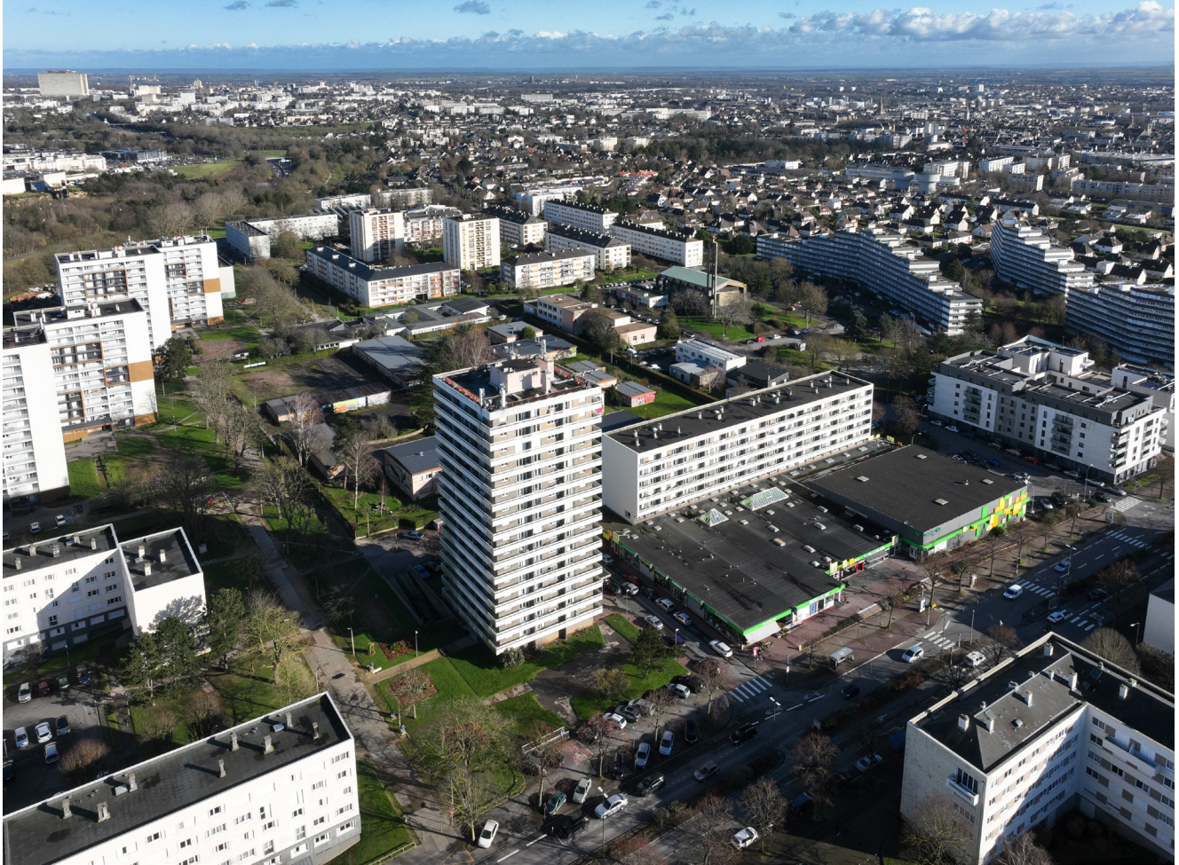
GENERAL AERIAL VIEW OF THE PROJECT SITE IN THE STUDY SITE
