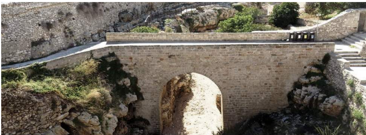
The remains of Trajan's Bridge
