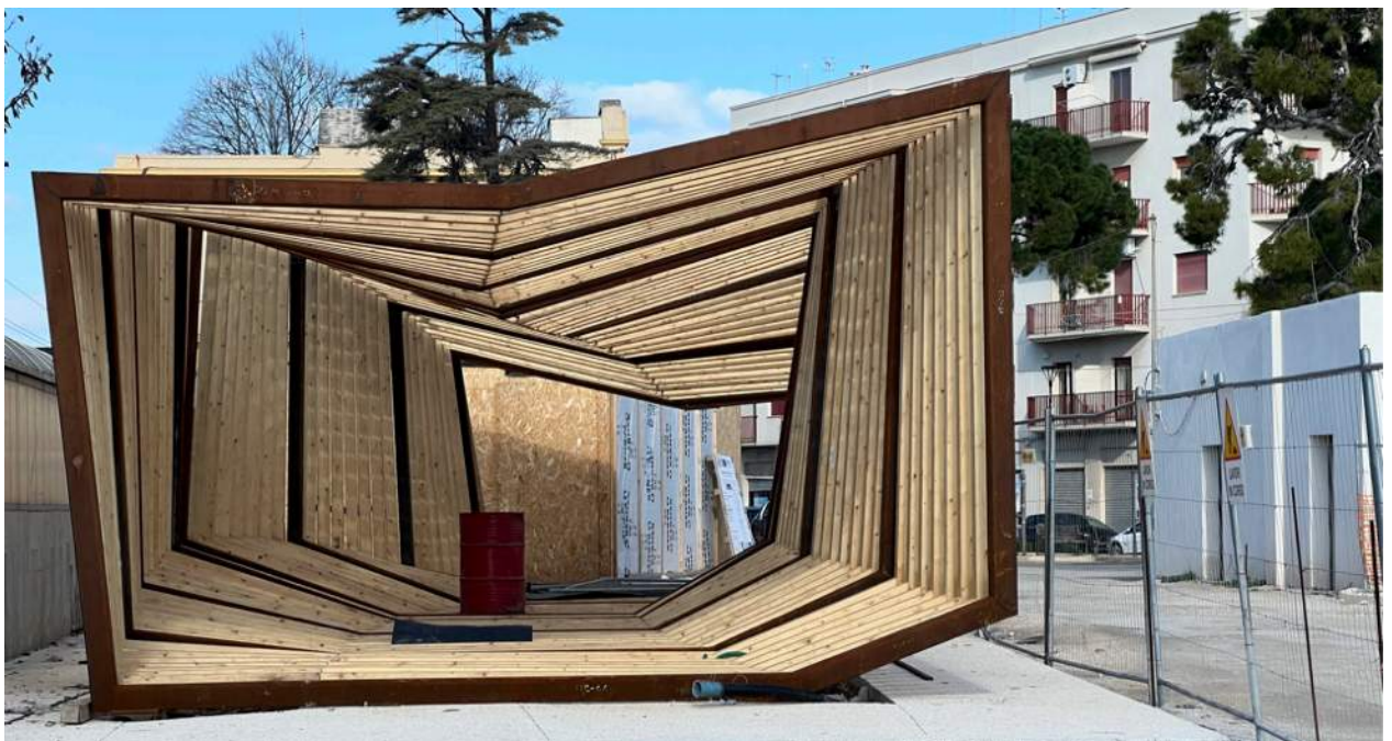
Velostation project nearing completion
