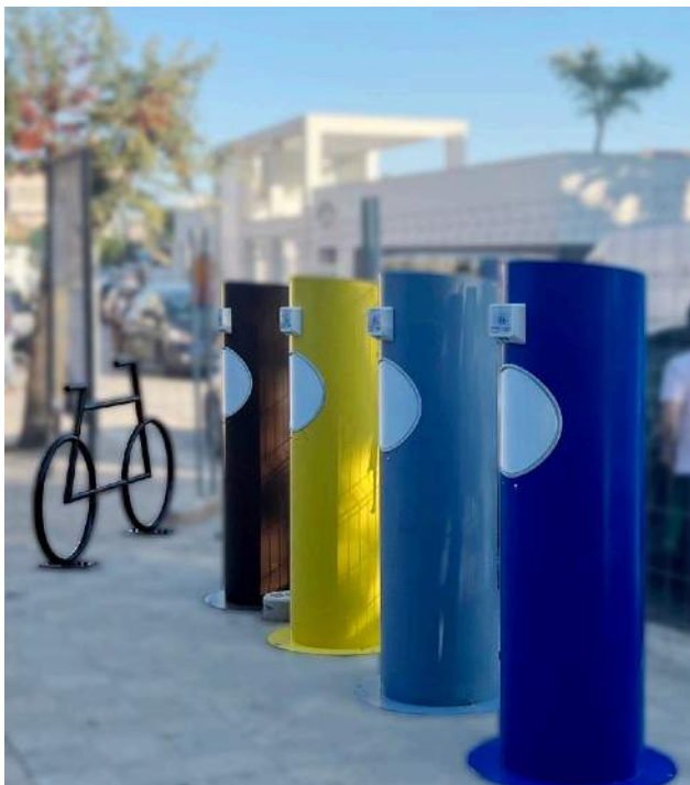
New pneumatic waste collection system - under testing
