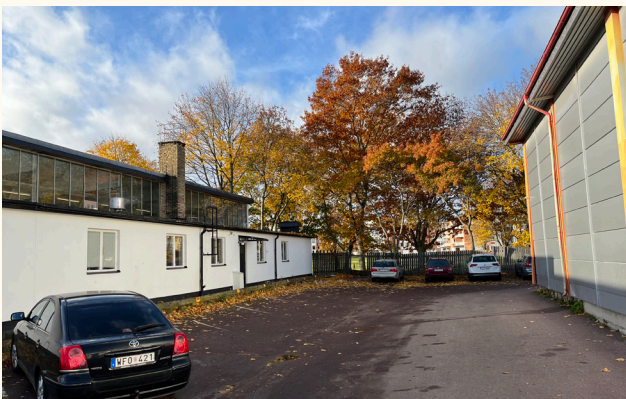
Buildings in Blockgatan. Photo: Karlstad Municipality
