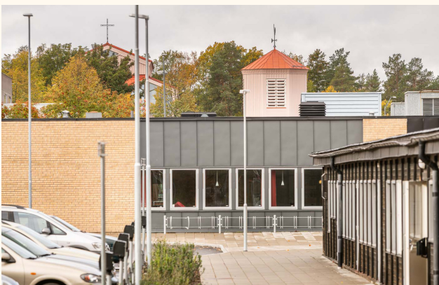
Building to be demolished or dismantled.
