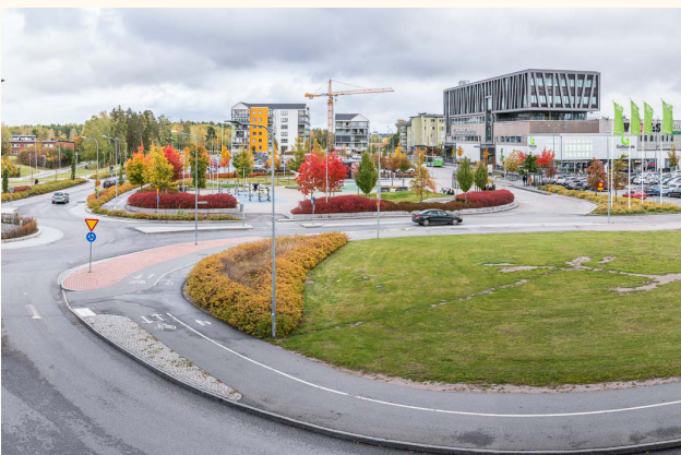
View of the roundabout.
