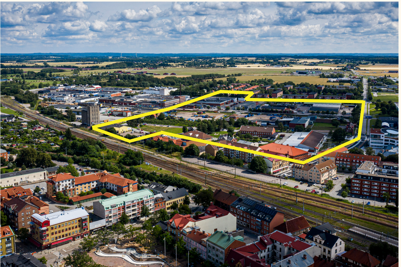
Eslöv with the project site on the eastern side of the railway. Photo by Christoffer Borg Mattisson
