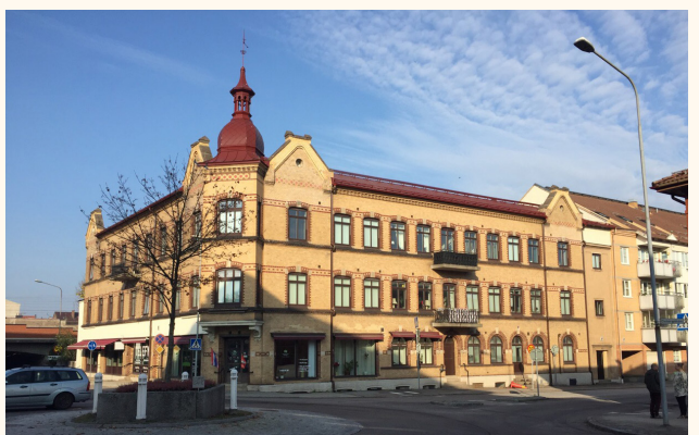
8. A former grocery shop (1899).
