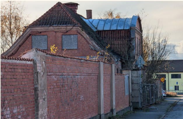
The brick wall.
