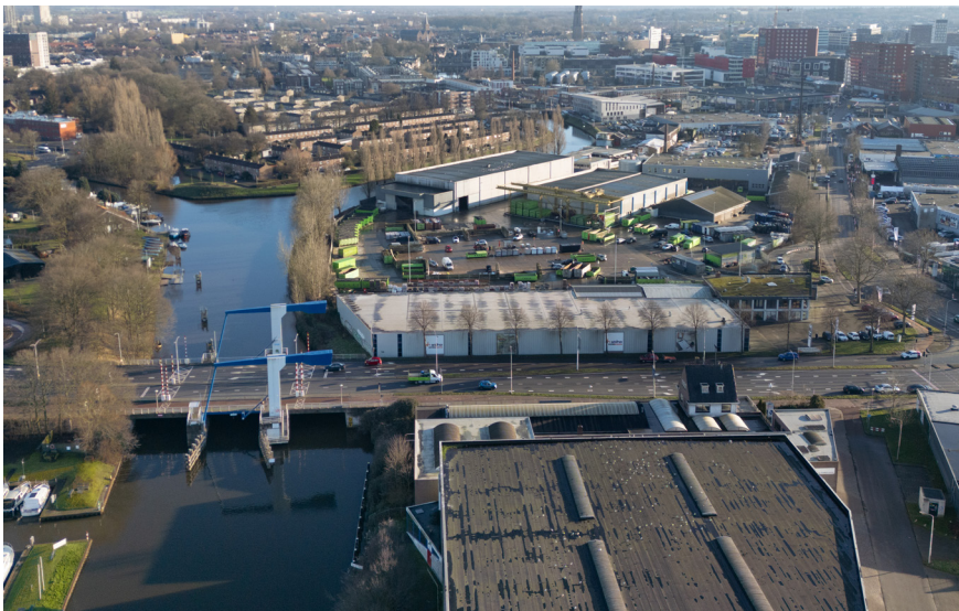
Aerial View of Koppelbrug
